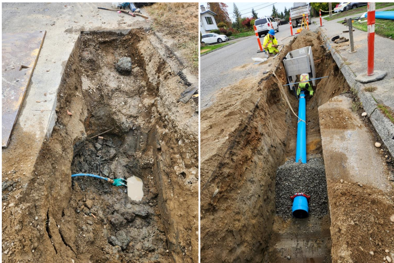
IMAGE | ROYAL ST. LOOP PROJECT – LEFT: SERVICE LINE CONNECTION; RIGHT: 250-MM BIONAX® PIPE.
