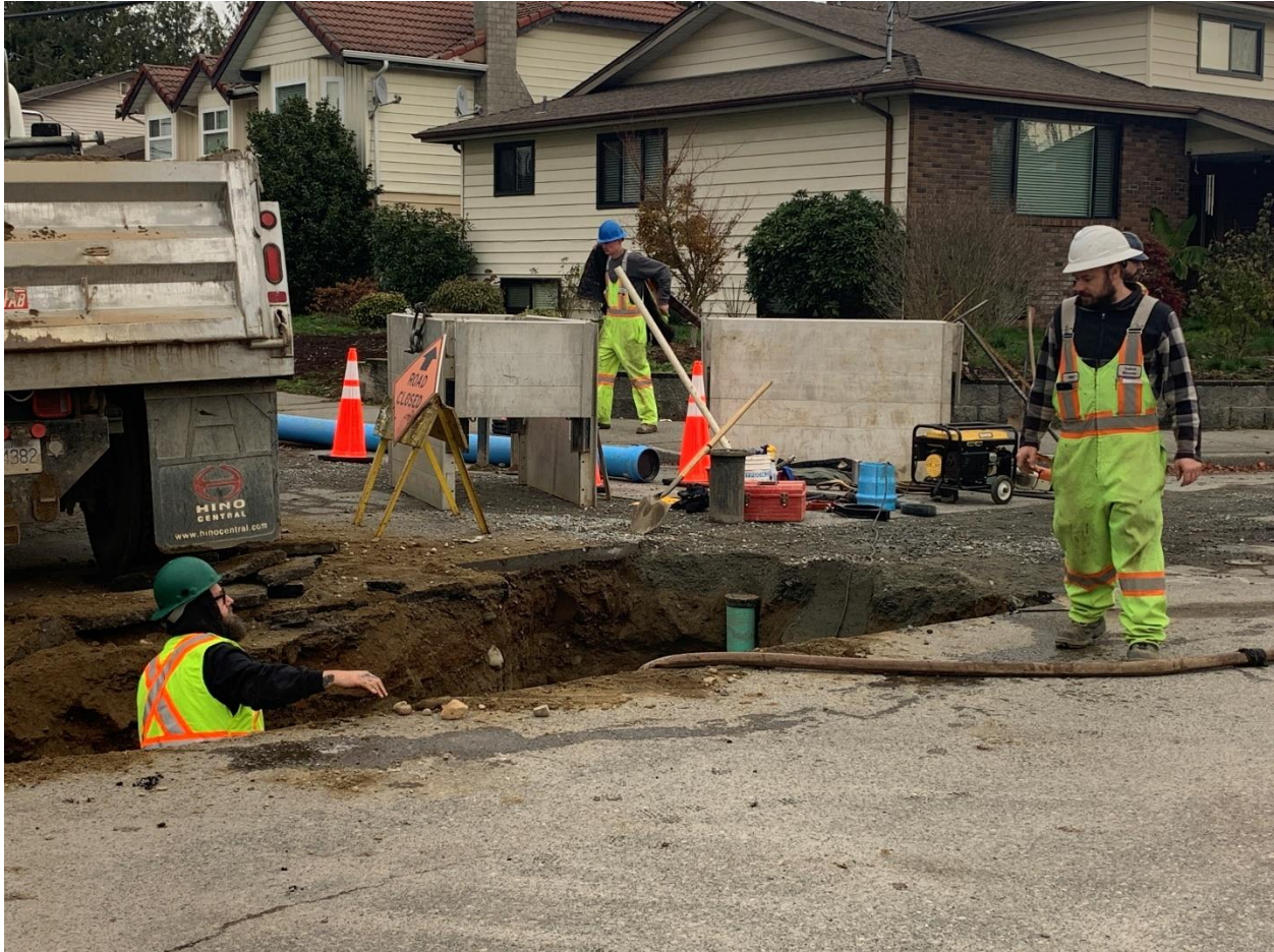
IMAGE | ROYAL STREET WATER MAIN LOOP PROJECT, COMPLETED IN-HOUSE.
