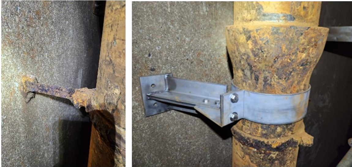
IMAGE | LEFT: ORIGINAL BRACKER; RIGHT: NEWLY INSTALLED STEENLESS-STEEL BRACKET.
