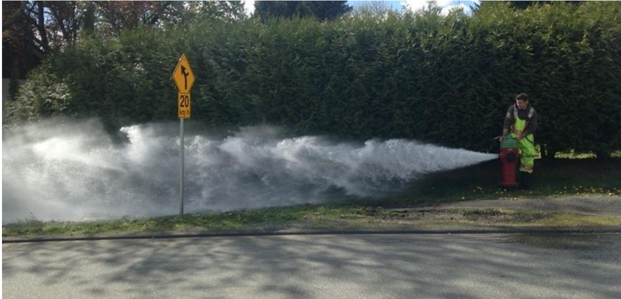
IMAGE | WATER SYSTEM FLUSHING IN PROGRESS.
