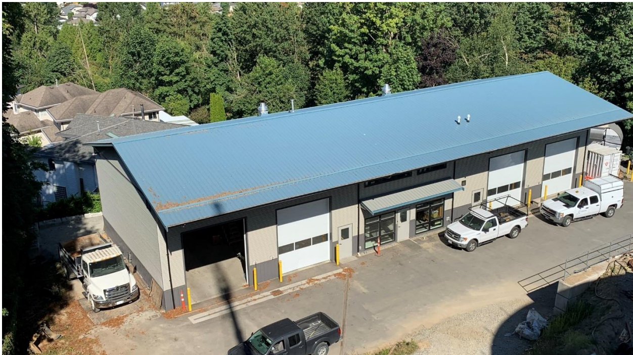
IMAGE | CWD’S OFFICE & WORKS YARD (RESERVOIR SITE) AT 2889 GRANDVIEW CRESCENT.
