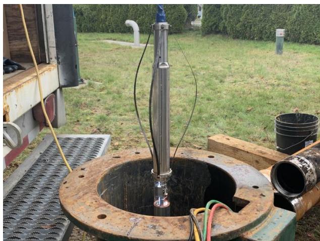
IMAGE | LEFT: THE DOWNHOLE VIDEO INSPECTION CAMERA; RIGHT: A SPECIAL WELL BRUSH USED FOR MECHANICAL AGITATION OF THE INTERIOR SURFACES OF THE WELL, PRIMARILY TARGETING THE SCREENED SECTION
