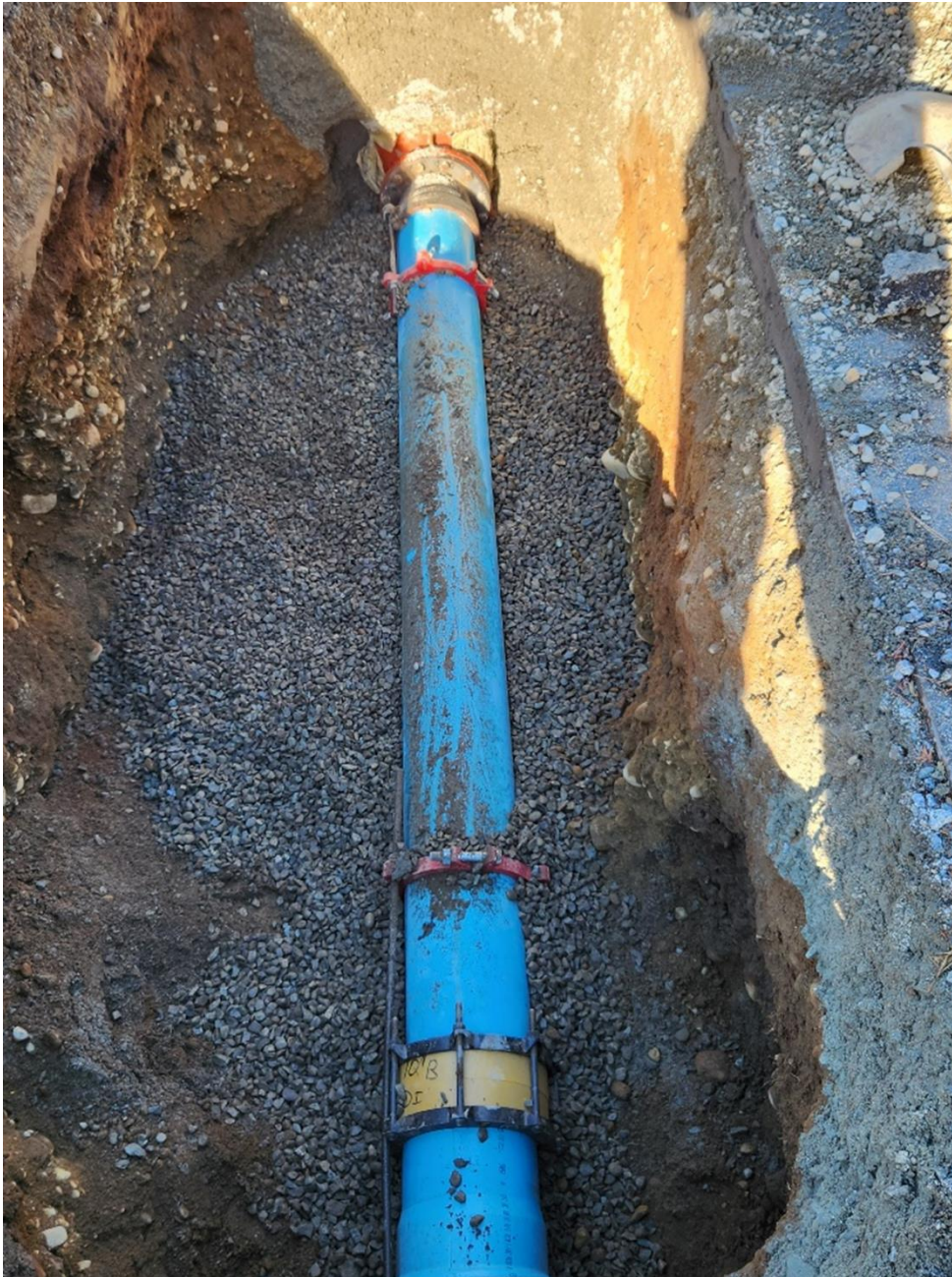
IMAGE | ROYAL ST. LOOP PROJECT –250-MM BIONAX® PIPE.
