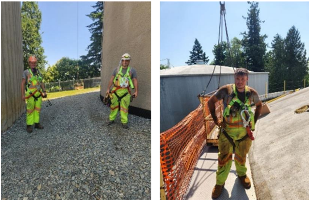
IMAGE | SPECIALY GEAR NEEDED TO SAFELY DECENT AND UNDERTAKE WORK IN THE RESERVOIR.
