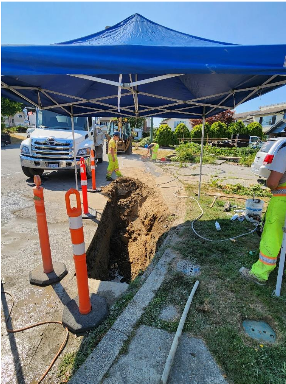
IMAGE | ROYAL STREET WATER MAIN LOOP PROJECT, COMPLETED IN-HOUSE.
